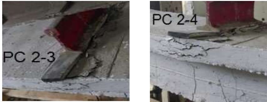
Fig.7: Mode of failure of the girders (PC 2-1, PC 2-2, PC 2-3and PC 2-4)
